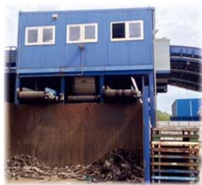
Ventilation & Venting for Sorting Cabins
